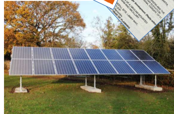
Typical "Ballasted" construction example No penetrative fixings allowed on the landfill cap
